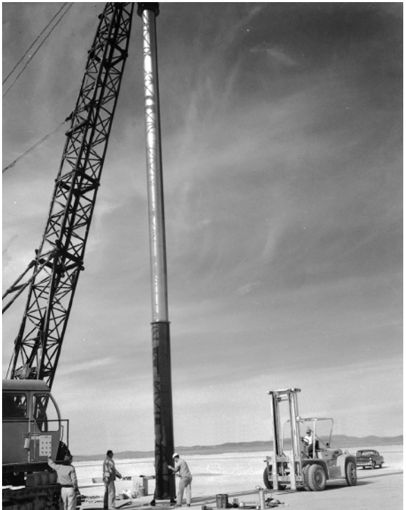
Setting up the legendary Area 51 pylon, or radar test pole. The radar antennas, manned and monitored by EG&G, were located a mile away from the pole. (Collection of Roadrunners Internationale/CIA)
