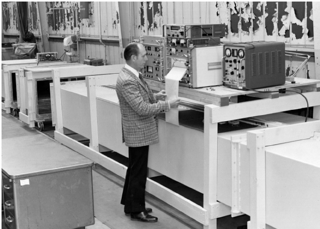
Ed Lovick, at Skunk Works in the mid-1960s, with the waveguide, as he works to reduce the radar cross section for the A-12 to meet the CIA's demands. (Collection of Edward Lovick/Lockheed Martin)
