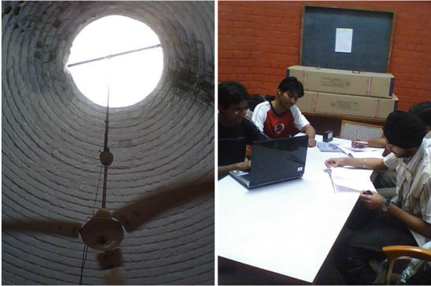
Fig. 2.6 Skylight components (SC) in experimental dome-shaped mud house for working place at the centre of floor at IIT Delhi
