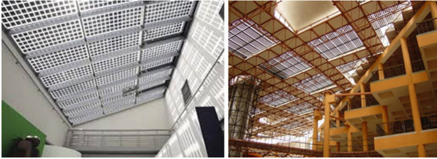
Fig. 2.9 View of roof-integrated semitransparent photovoltaic (PV) module
