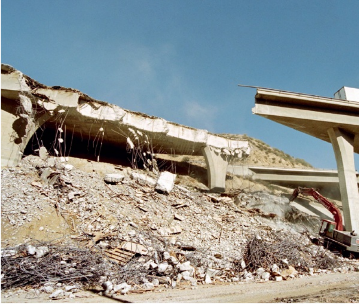
A portion of highway 5 in California collapsed after a magnitude 6.7 earthquake hit outside of Los Angeles in 1994.
